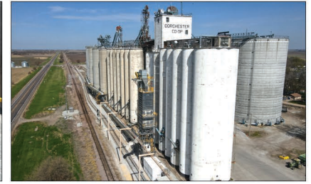
The system monitors high & mid-level sensors in the bulk weigher w/70,000 bu./hr capacity.
